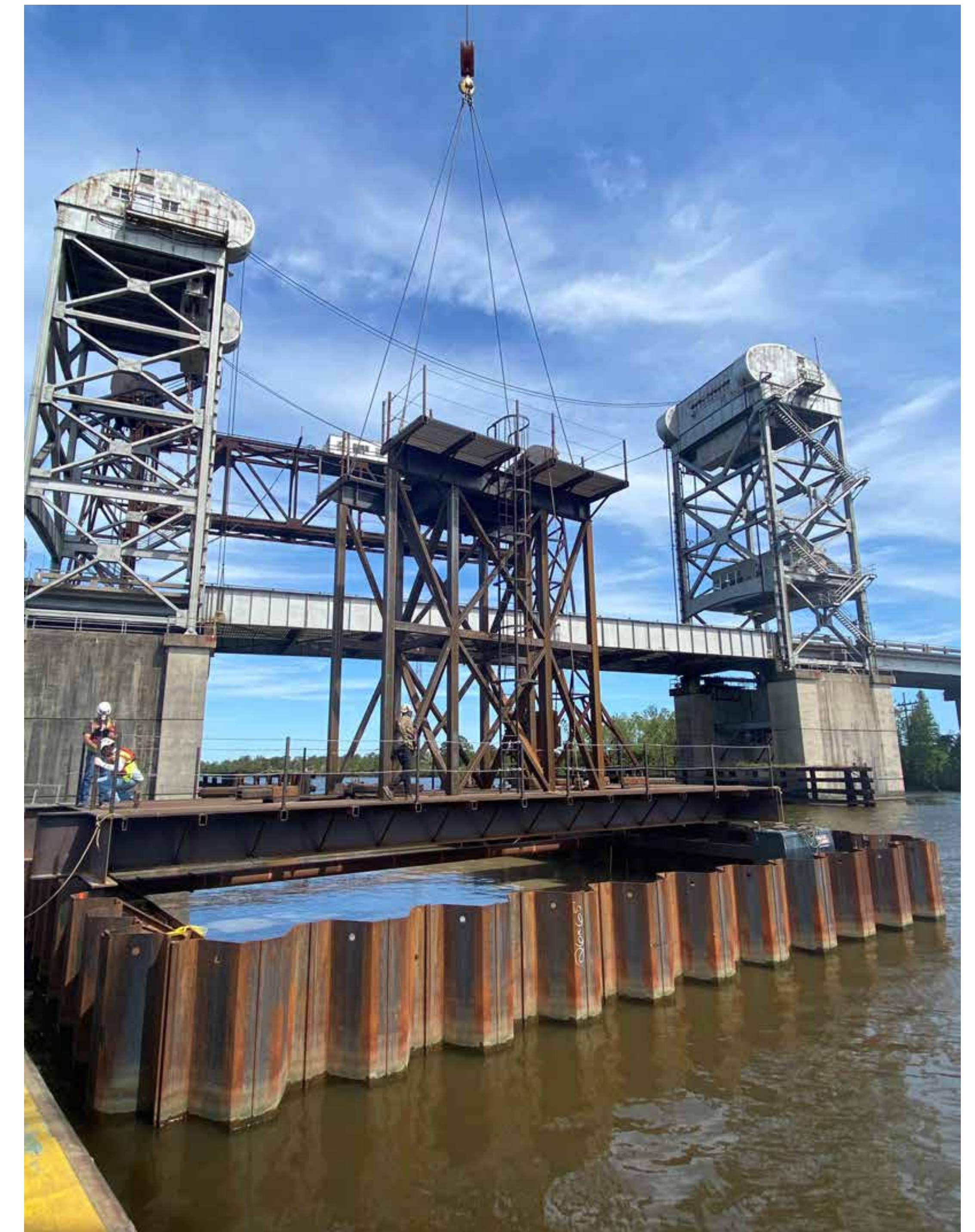
Main Pier 1 Setting Battered Pile Template
