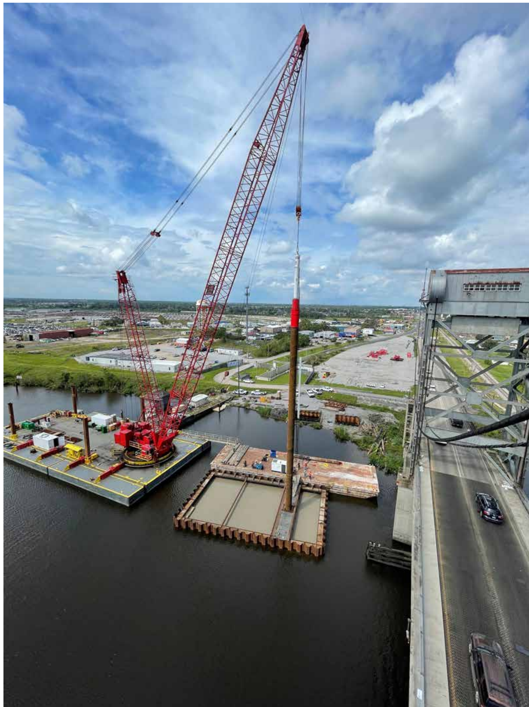
Driving First 48" Pipe Pile at Main Pier 1
