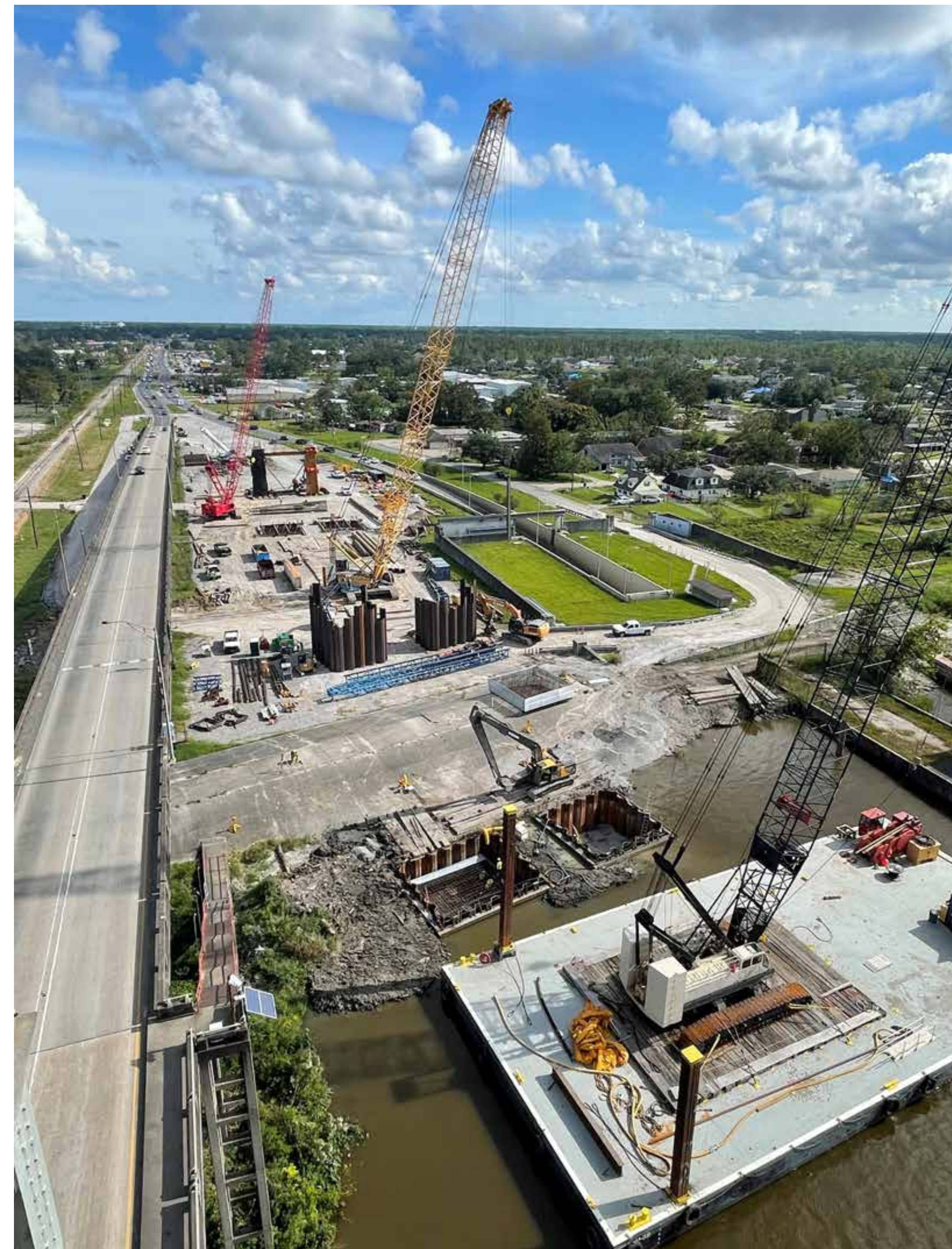
South Side Progress with cofferdams, footings, and columns shown
